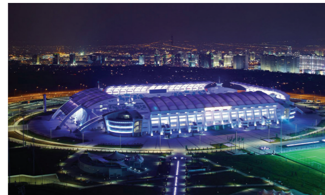
Project: Asian Olympics Stadium Project / Projekt: Asian Olympics Stadium Projekt
