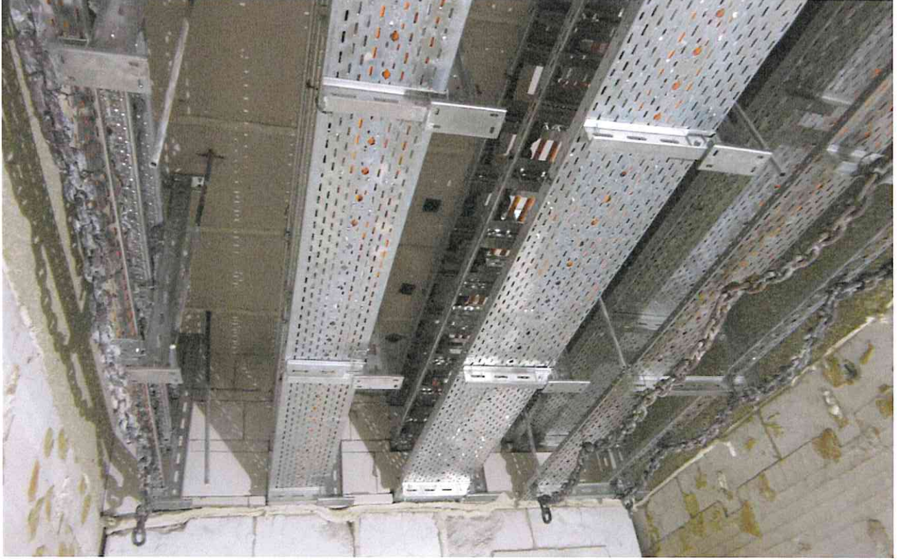
Photo B1: Test setup of the cable system before the test
