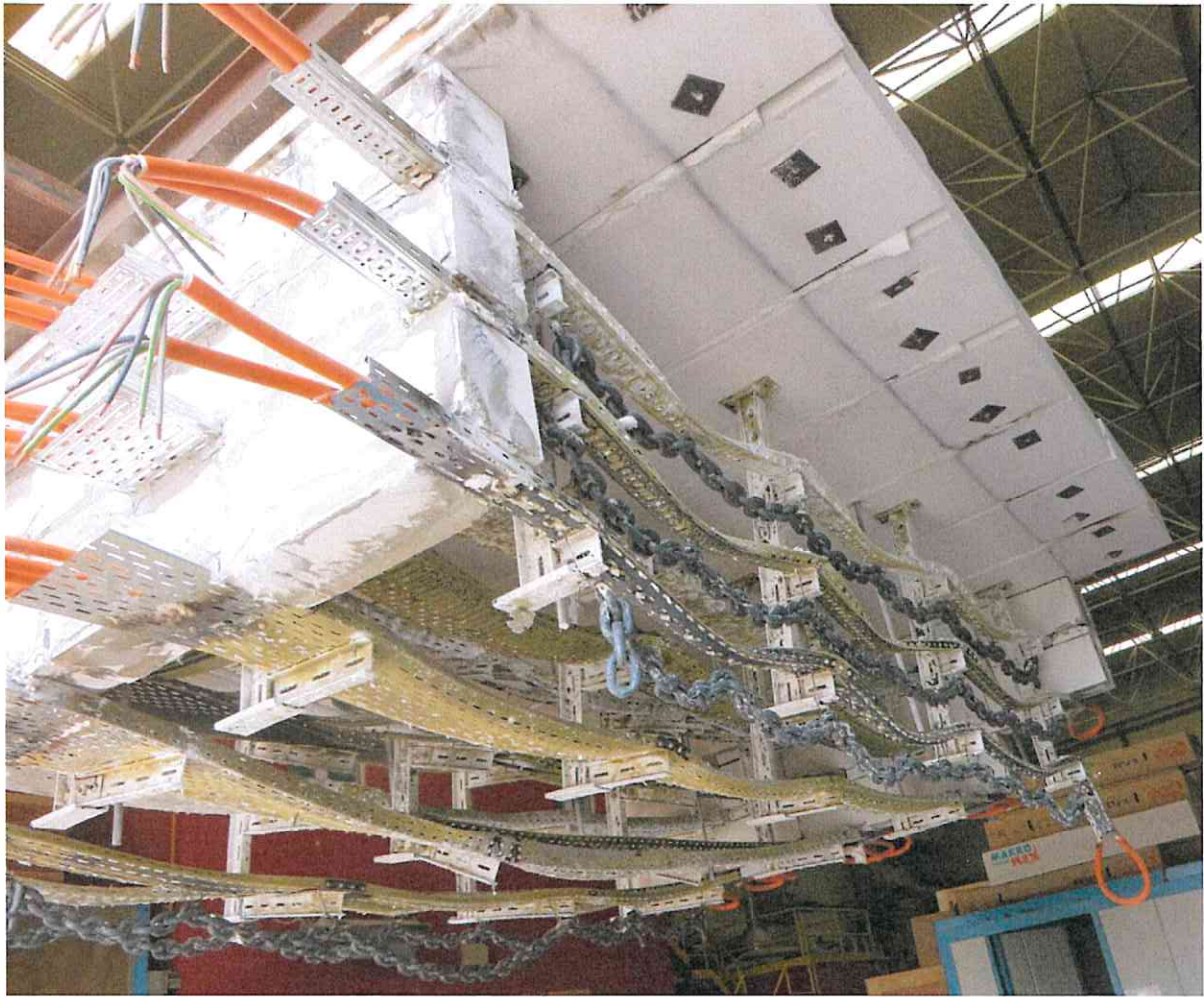
Photo B2: Exposed side of the test specimen after the test
